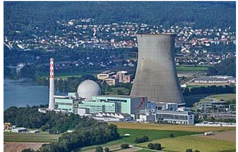
Leibstadt NPP, Switzerland. BWR Nameplate capacity 1,220MW, Capacity factor 87.6%.
