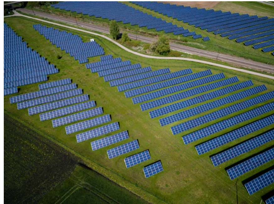
Utility Solar – PV arrays
