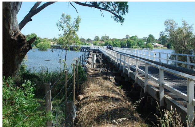
Kirwans Bridge (310 metres long) opened in 1890 and still used today
